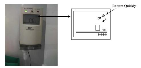
On the HF detector verify that it is powered up and no trouble light or alarm are present. Verify the sampling pump is rotating. If the pump is not rotating the trouble light will Become yellow. Notify staff.
