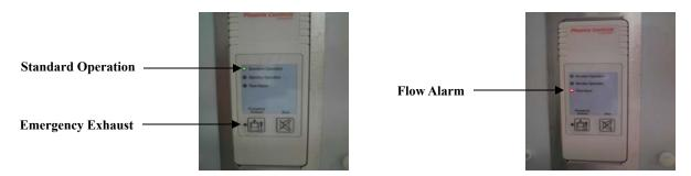
If no alarms on the HF detector are found verify the Phoenix controller standard operation LED Is lite. This indicates the exhaust is at the proper flow rate. If the standard operation LED is off And the flow alarm is on and alarming push the emergency exhaust then lower the bench sash and notify staff immediately. If no alarms continue with your task.
