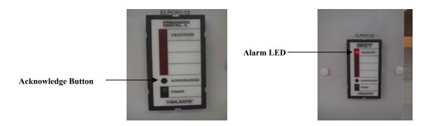
Verify the precision digital controller is powered on. The controller is used to inform you when the sash is out of position.
